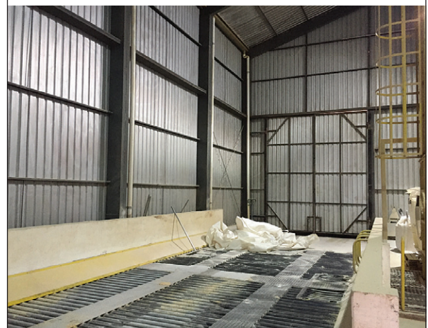
FIGURE 19 Closed hopper that avoids the entry of birds
